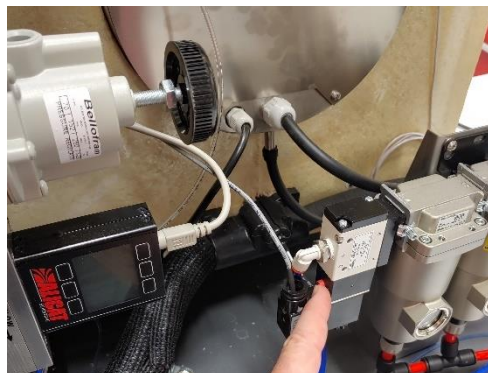
Figure 3.9B Red Button on Air Dryer Solenoid
